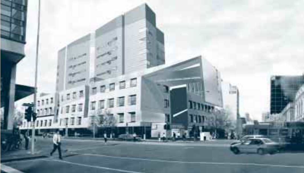
An artist's impression of the Victorian County Court. It is expected to be completed mid-2002.
