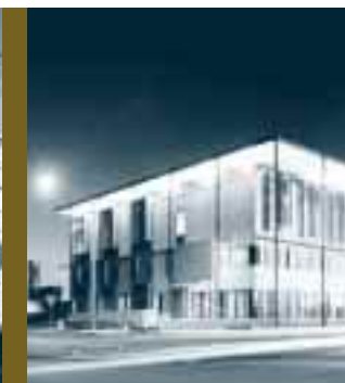
The Ballarat Police Station and Law Courts
