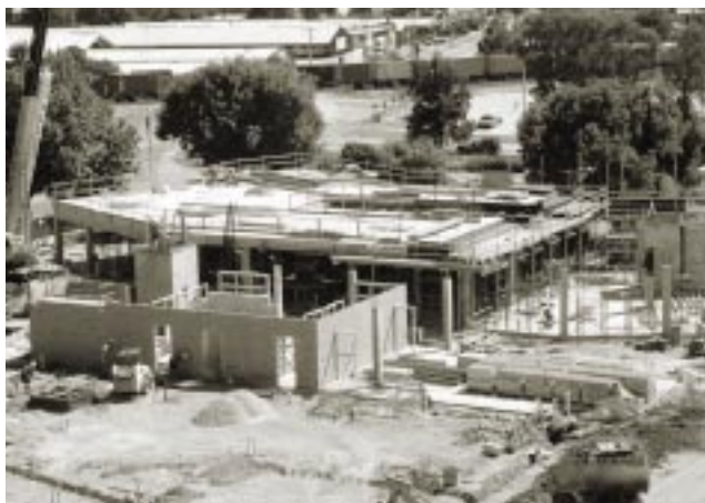
The Wodonga Police and Courts Complex – ready for use in 2002.
