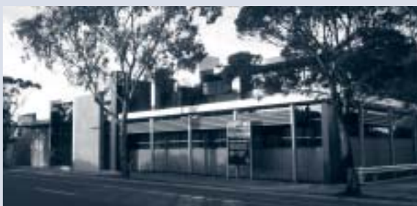
The $6.44 million Northcote Police Station is part of the State Government's $280 million program to improve and upgrade police stations across Victoria to house a record number of police.
